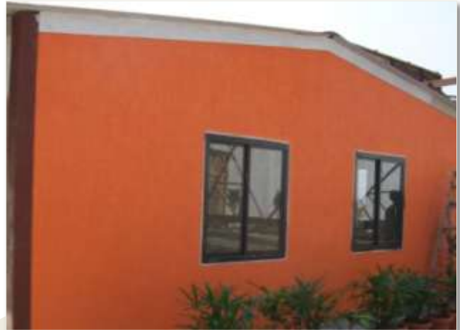
Exterior paint / texture finish
